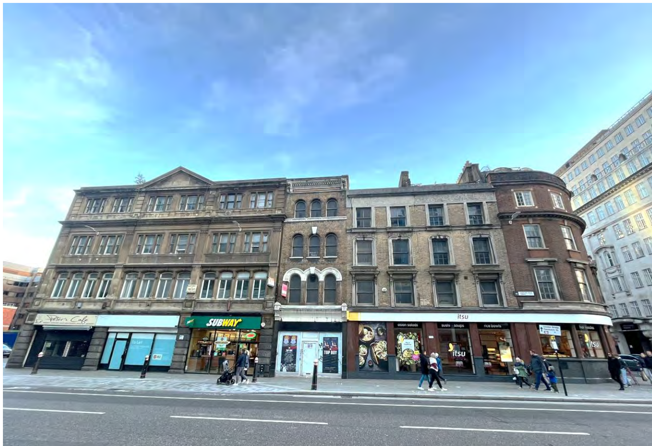
The Victorian terrace along the south side of Aldgate High Street (73-78) with Minories to the right side (Credit: SAVE Britain's Heritage)
