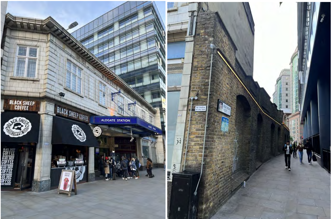
Left: The 1926 frontage to the unlisted Aldgate Underground Station | Right: Blue Boar Alley looking north, which would form the eastern boundary of the expanded Conservation Area proposed by SAVE and others (Option 3 Plus) (Credit: SAVE Britain's Heritage)
